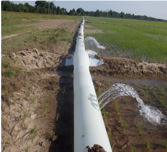
Fig. 1. Multiple inlet irrigation is required when implementing AWD.
